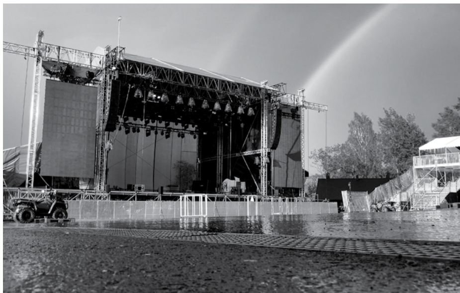
Photo: LT Roof, Aku's Factory, Finland
