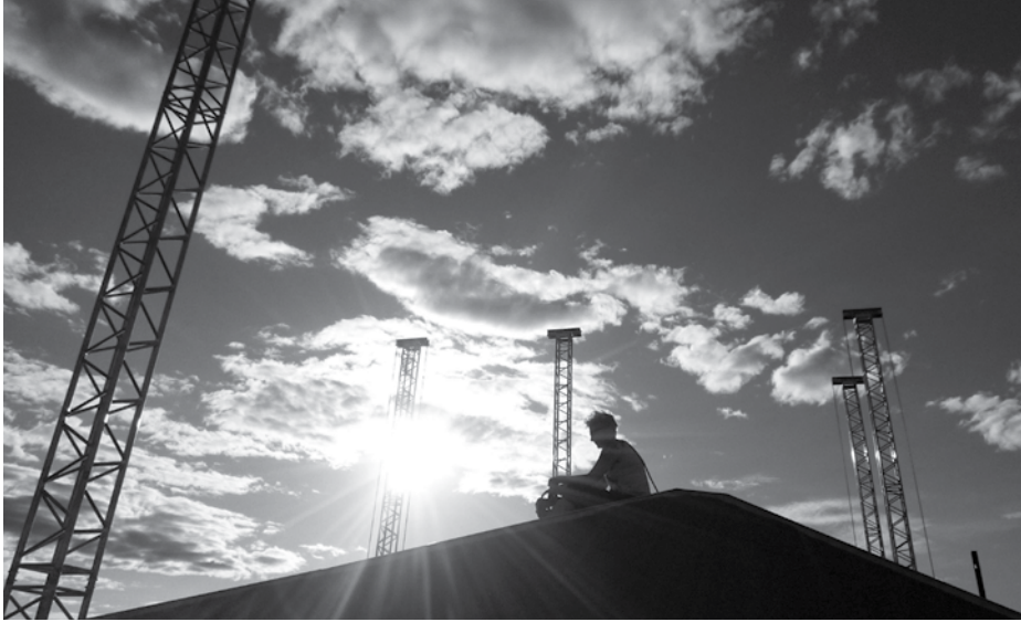
Photo: LT Roof, Aku's Factory, Finland
