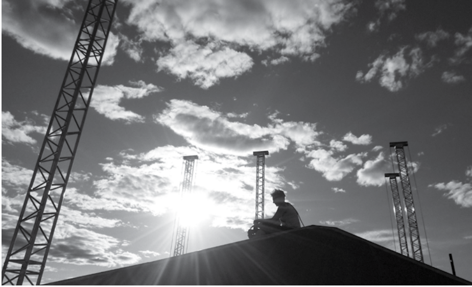
Photo: LT Roof, Aku's Factory, Finland
